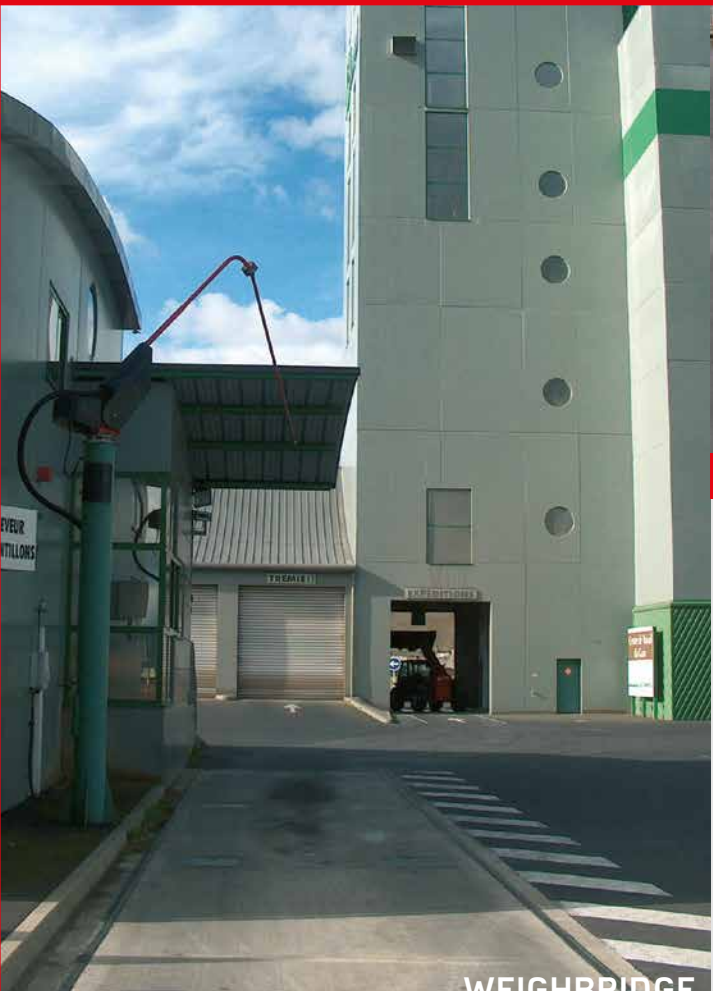
WEIGHBRIDGE HANDLING TRUCK INPUT/OUTPUT
